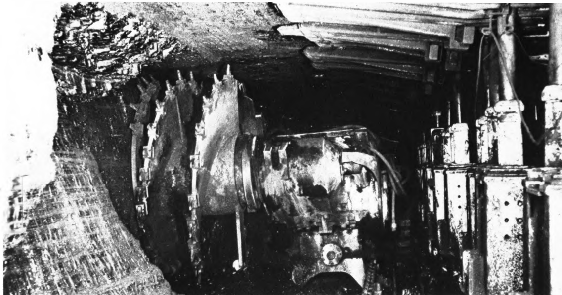
44 An electrically driven continuous mining machine operating in an American mine. The Americans pioneered the use of such machinery in the late 1940s
